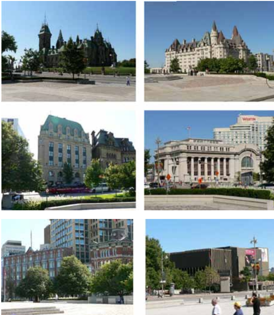
Figure 10. Confederation Square National Historic Site, which rings the War Memorial. Clockwise from top left: East Block, Parliament Hill; Chateau Laurier Hotel; Union Station; National Arts Centre; Central Chambers, Bell Block and Scottish-Ontario Chambers; Central Post Office and Langevin Block. (Photographs by author)
