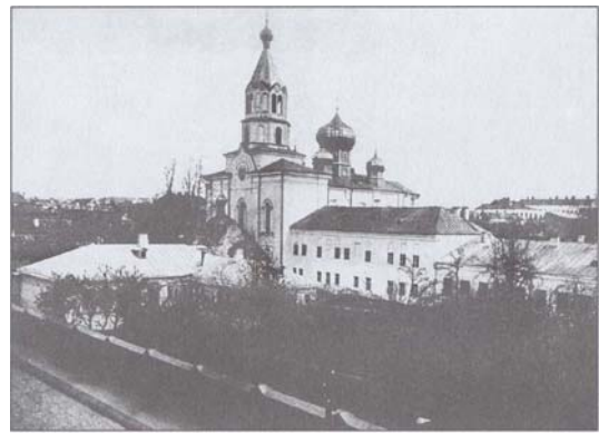
The view of the Benedictines Cloister after rebuilding of its original structure to "the true Russian style" in 1870
