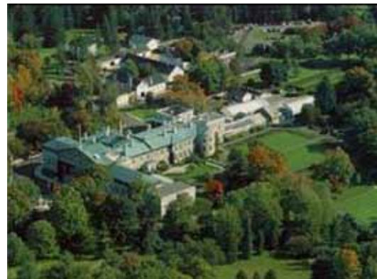
Figure 3. Aerial view of Rideau Hall showing residence and immediate surroundings.
