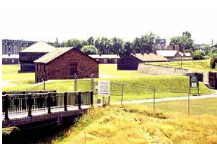
War of 1812 Buildings at Fort York
