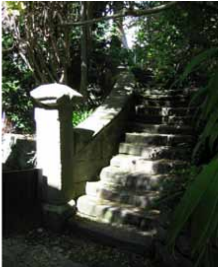
Remnants of the estate garden remain among the 1930s and 40s apartments
