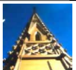
Copper work at St. Michael's Cathedral
