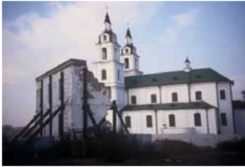
Historical building, destroyed in 1996 without reasons.
