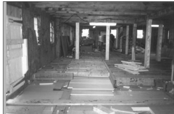
Figure 4. Conservation work on the Depot in the 1990s.Elements of the foundation were repaired and replaced, insulation was placed beneath the floor to stabilize the permafrost, and drainage was improved.(photo from Parks Canada)
